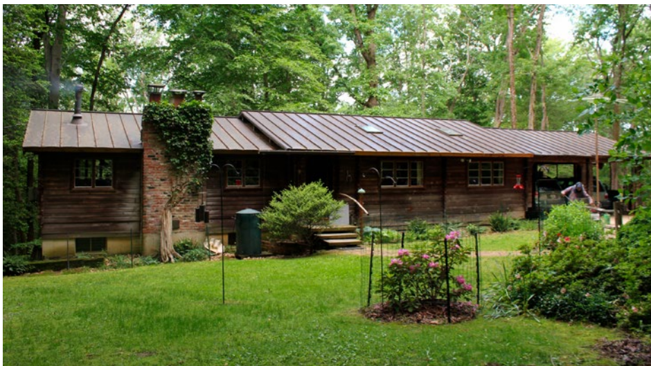
The KOCH HOUSE (opposite page) located on Overlook Drive in Poplar Hill was designed by Harold Esten, who studied architecture at the Illinois Institute of Technology in Chicago and opened a practice in Silver Spring in the 1950s. Credit: Dave Koch
